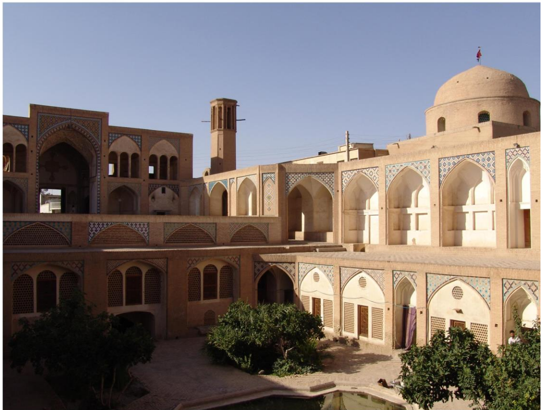
Agha Mosque City of Kashan Photographed by Khosrow Bozorgi
